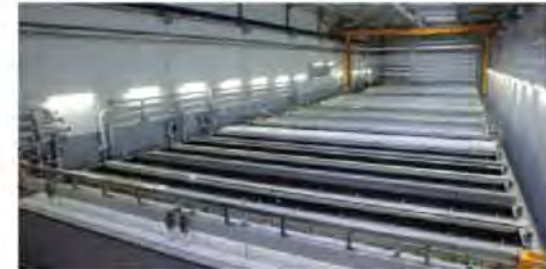
Anodizing plant – technological tanks to bath
