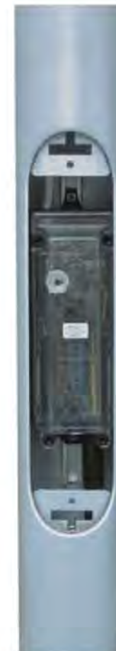
Connection box Installed in aluminium column
