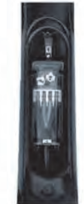
wiring chamber in pole SP
