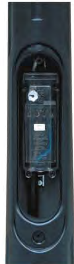
Connection box installed In plastic coated pole
