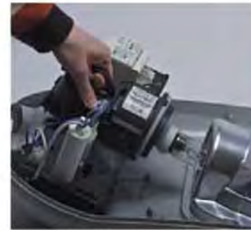
Removal of control gear to facilitate lamp change without moving optic ⤴
