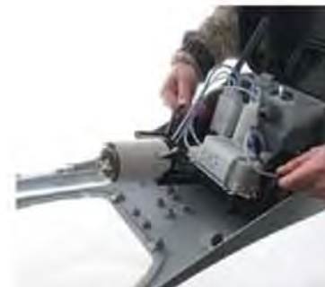
Removal of control gear \uparrow
