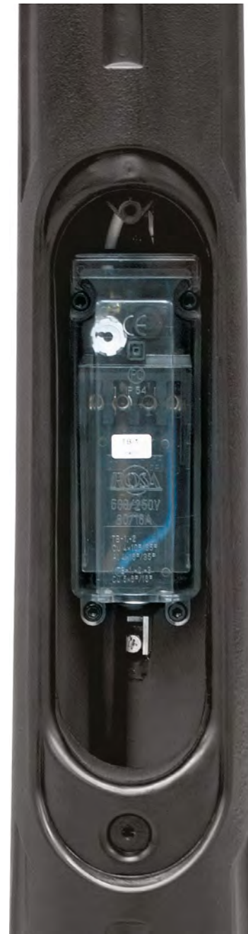
Connection box installed in plastic coated pole
