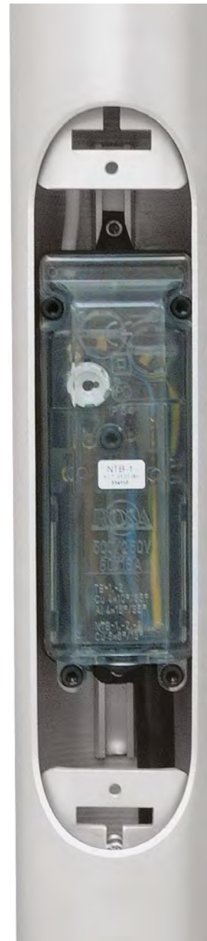
Connection box installed in aluminium column
